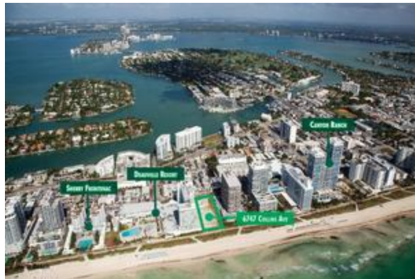
China City Construction Co. acquired the site at 6747 Collins Ave. in Miami Beach.
